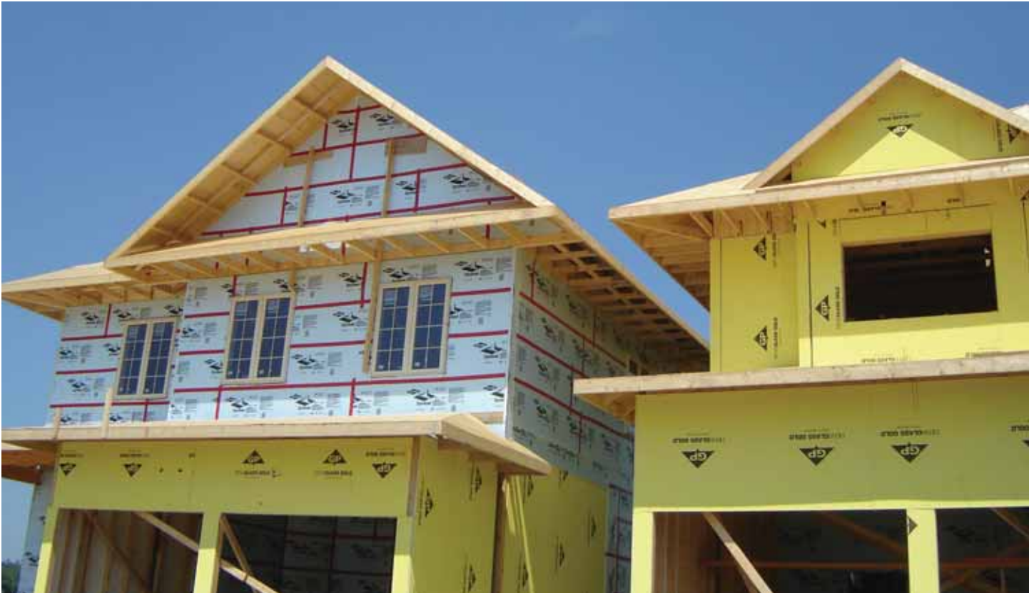
Top picture: house construction showing the deep overhangs Bottom picture: cistern used for rain harvesting
